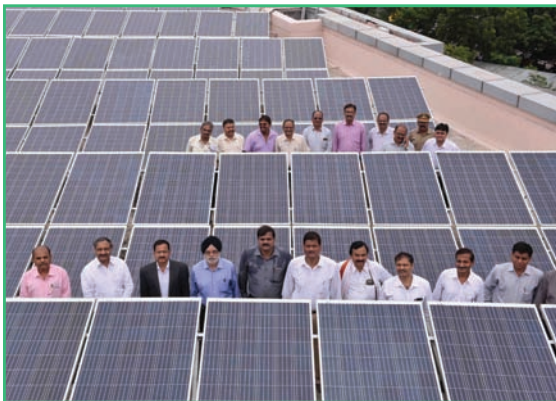
Installation of Solar Panels at MOIL Head Office
