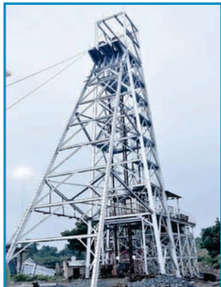
Second Vertical Shaft at MOIL's Chikla mine
