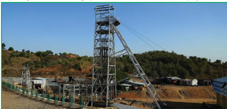
Vertical Shaft at Munsar Mine
