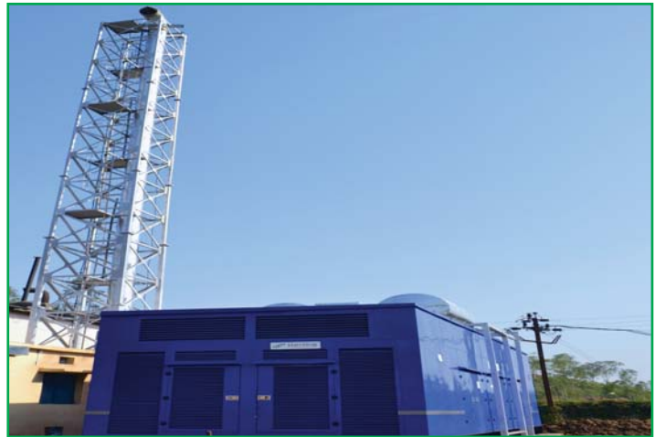
Generator installed at MOIL's Balaghat Mine
