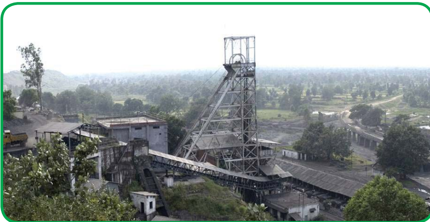
VERTICAL SHAFT AT BALAGHAT MINE
