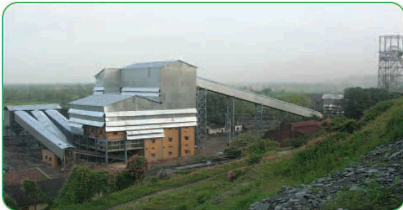
MOIL'S INTEGRATED MANGANESE BENEFICIATION PLANT OF 500000 TPA CAPACITY AT BALAGHAT
