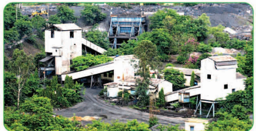
MOIL'S INTEGRATED MANGANESE BENEFICIATION PLANT OF 400000 TPA CAPACITY AT DONGRI BUZURG
