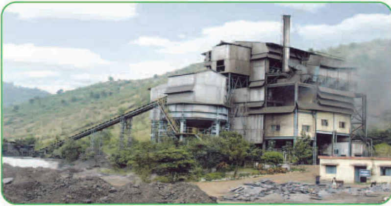
MOIL'S FERRO MANGANESE PLANT OF 10000 TPA CAPACITY AT BALAGHAT
